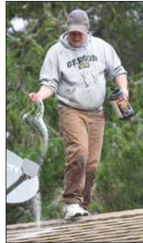
Treat mossy roofs with granular moss killer, or a liquid mixture sprayed on the offending greenery.
