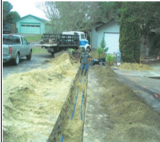
The pictures above show the water service replacements being done in Greentrees Village. The top left photo shows the road being excavated; top right shows the new 'saddle' being connected to the water main. The bottom left photo shows the new water lines being placed in the road and in the bottom right photo, a worker holds up the old saddle to show the corrosion inside the orifice. A new water service box is in the background.
