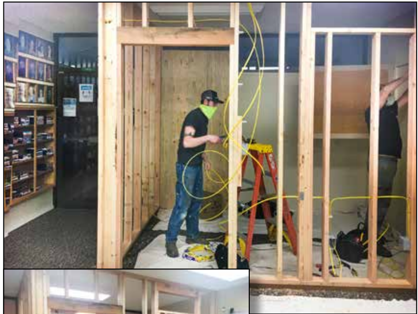
Electricians from Lighthouse Electrical Contractors run wiring for lights, phone lines, cable, and internet in what will be the official GTV General Manager's office. -- Photos by Laurie White
