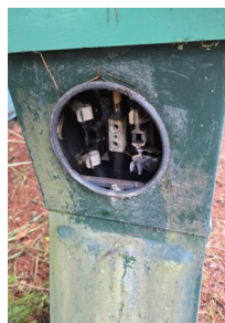
Electric pedestal corrosion from dampness heat salt air
