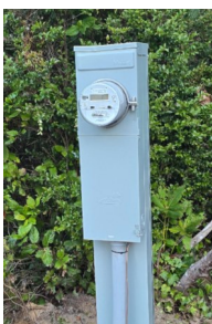
New electrical pedestal—height is approximately 5 feet at top
