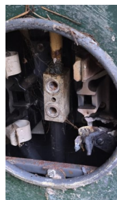
Electric pedestal corrosion from dampness heat salt air
